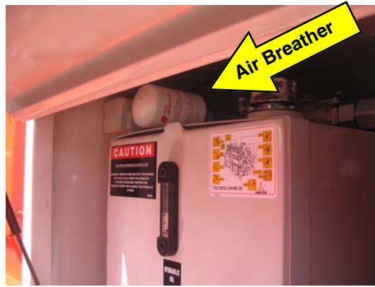
Checking/ Changing Hydraulic Tank Air Breather HF4003
