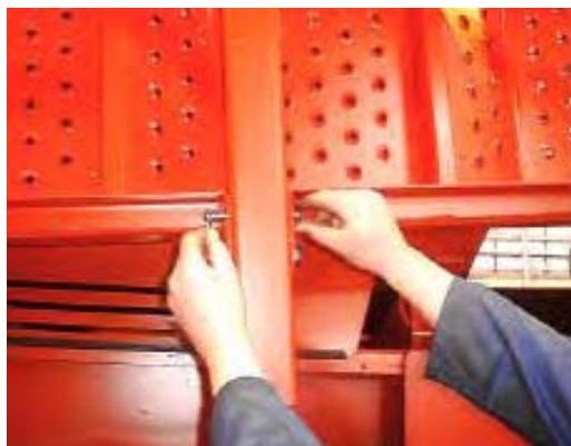
1: Remove R-clips & handrail retention pins.
